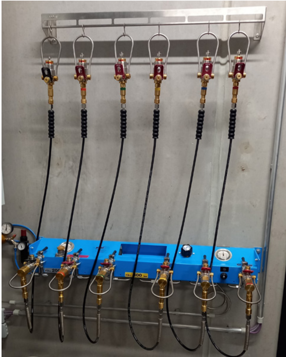
Filling breathing air cylinders with WEH® connector TW154.
